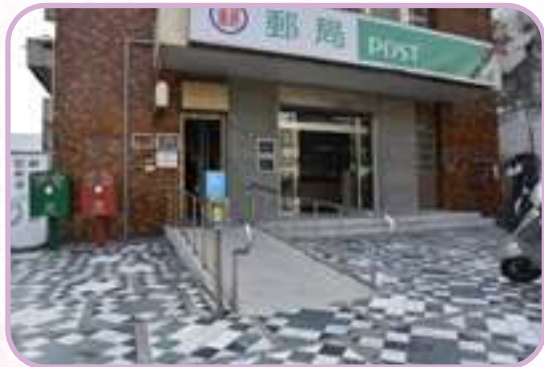
Accessible Facilities and Service Bell
